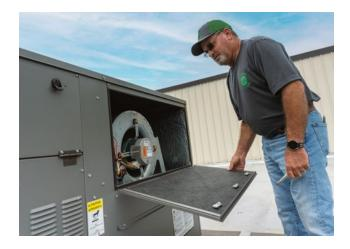
Rheem HumidiDry uses an additional reheat coil inside the unit to achieve peak comfort. "When you cool air, moisture comes out of the air, but then it's too cold for occupants to be truly comfortable. You have to reheat the air," says Laura Meyerrose, Rheem Commercial product manager. "It goes over that heating coil to bring the air back up to comfortable heating levels."
